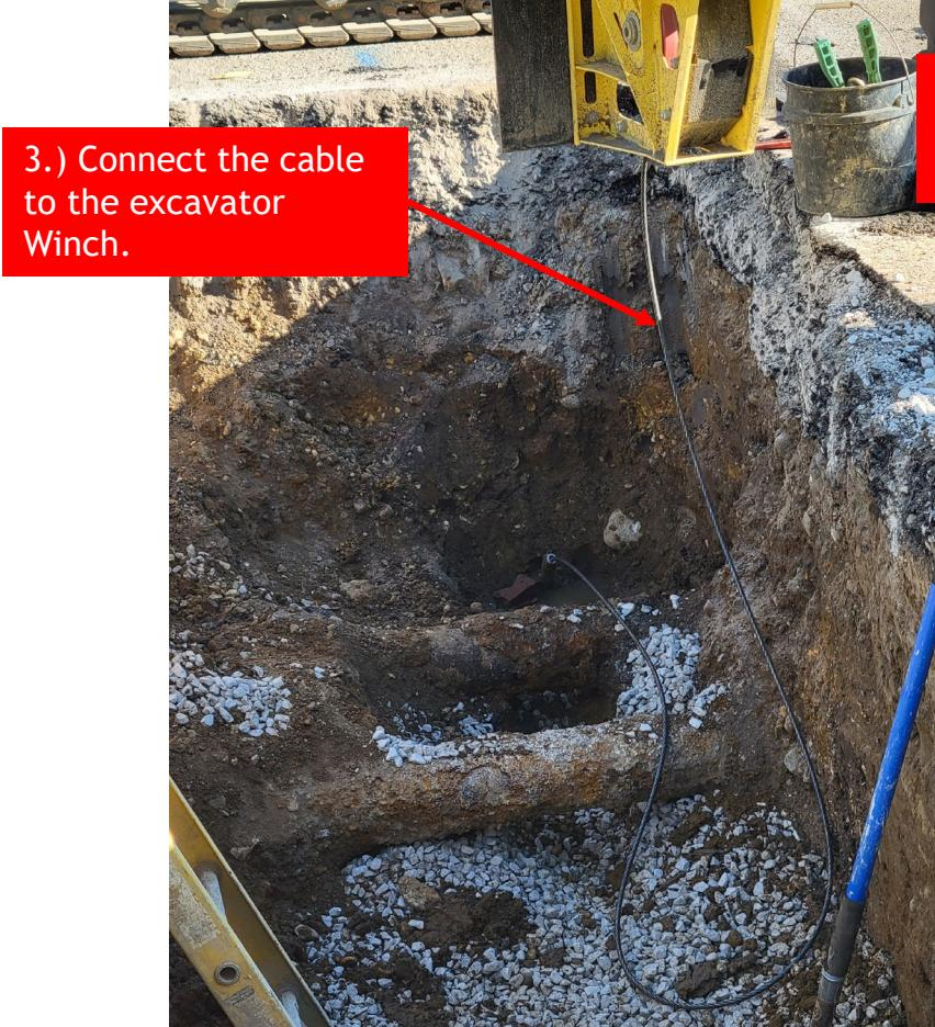
4.) Pull out the old service line, replacing it with the new line.
